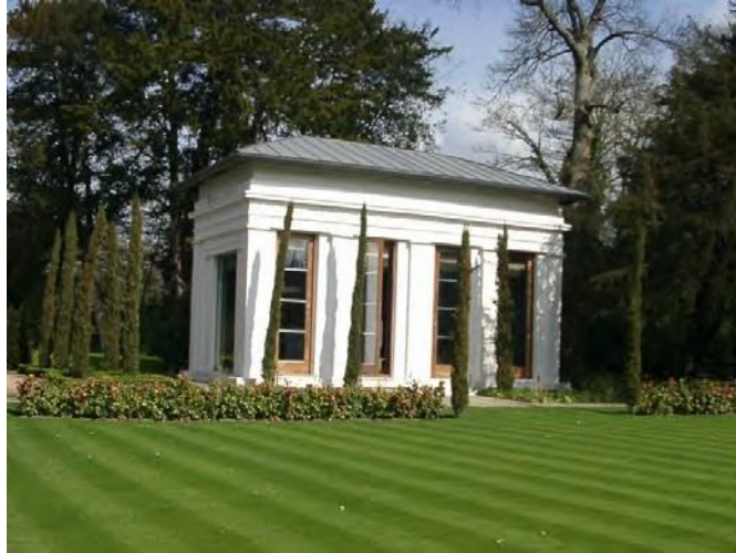
Picture 2.2 Ad Astra Orangery, Priory Drive, Stanmore
