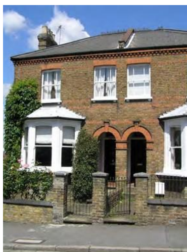
Picture 3.6 83 West Street, Harrow on the Hill
