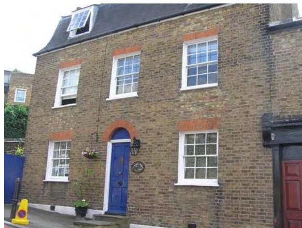
Picture 3.10 38 West Street, Harrow on the Hill
