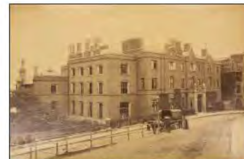
View of The Head Master's Boarding House (late C19)
