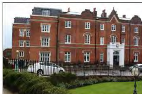
View of The Head Master's Boarding House (2012)
