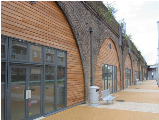
Figure 5.5 Business Use Railway Arches, Brember Road
