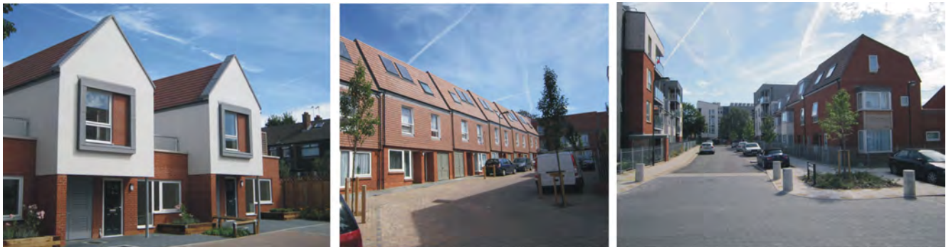
Picture 8 Rayners Lane Development
