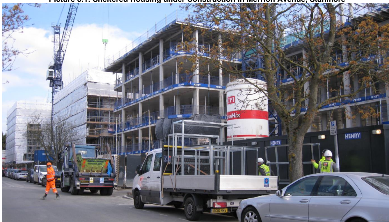
Picture 5.1: Sheltered Housing under Construction in Merrion Avenue, Stanmore
