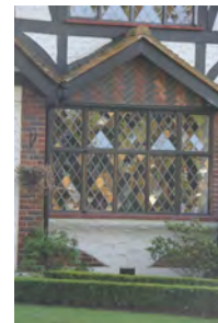
Picture 6.73 Timber/metal leaded light windows
