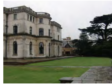
Picture 6.35 East Elevation
