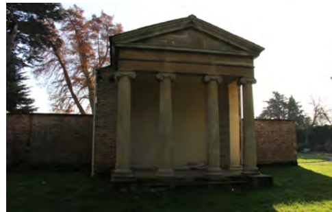
Picture 6.40 Garden Temple (North Elevation)
