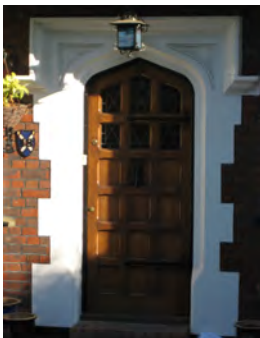
Picture 6.75 Pointed, heavy timber front door with good Tudor Revival doorcase detail
