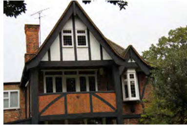
Picture 6.74 Tudor Revival style includes textured surfaces of contrasting materials and projecting and recessed parts give a three-dimensional character
