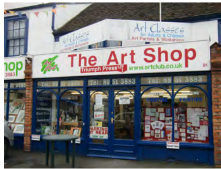
Picture 5.62 Use of modern fascia boards, stall risers and pilasters along Edgware High Street
