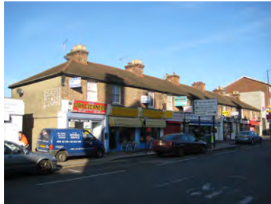
Picture 5.56 Nos. 1-12 Whitchurch Lane. A good Victorian terrace with their original timber sash windows
