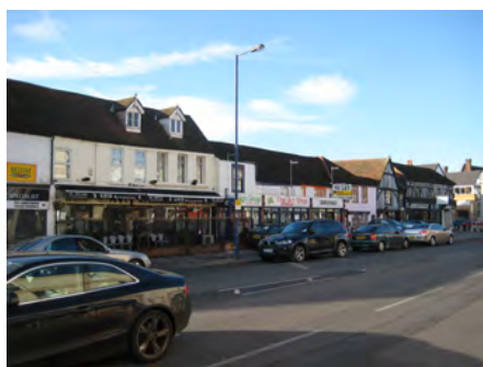
Picture 5.39 View of the High Street buildings nos. 85- 101 looking north - this illustrates their modest scale and design essentially as rural cottages
