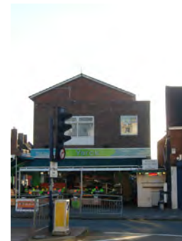
Picture 5.69 Railings around the corner of Edgware Road and Whitchurch Lane are damaged and add clutter to the streetscene
