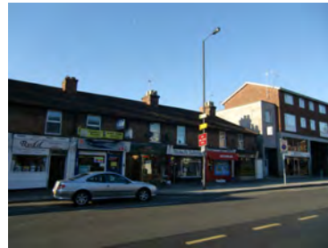
Picture 5.72 Abundance of street furniture and shop signage creates clutter within the streetscene along Whitchurch Lane
