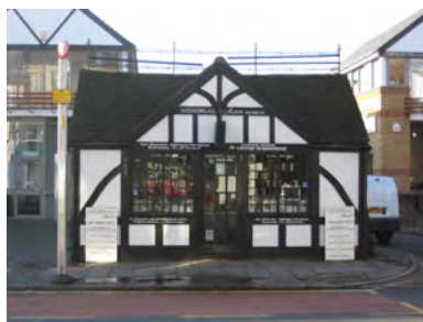
Picture 5.53 The positive unlisted Tudorbethan style no. 103 High Street, Edgware, with good metal railings above
