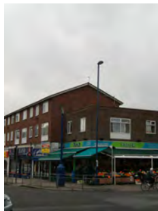
Picture 5.68 Street furniture clutter at the junction of Whitchurch Lane and Edgware High street
