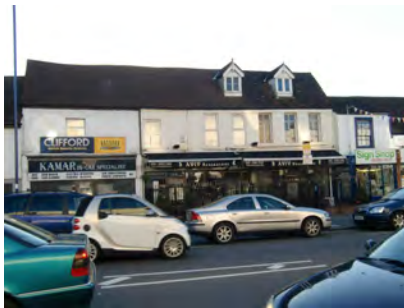
Picture 5.40 No. 85-89 High Street - likely to date to the 18th century with timber framing hidden behind render facing
