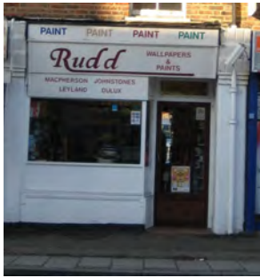
Picture 5.24 9 Whitchurch Lane- Typical original shopfront, with pilasters dividing it from its neighbour
