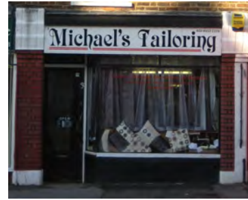
Picture 5.25 No. 12 Whitchurch Lane - good original shopfront with recessed entrance door
