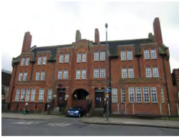
Picture 5.29 Locally Listed Police Station
