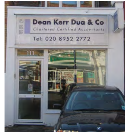
Picture 5.64 Shopfront to no. 111 does not preserve the character of the Conservation Area given UPVC and poor detailing
