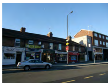
Picture 5.72 Abundance of street furniture and shop signage creates clutter within the streetscene along Whitchurch Lane
