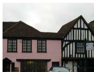
Picture 5.45 Unusual and complex roof structure nos. 95 and 97 High Street, Edgware
