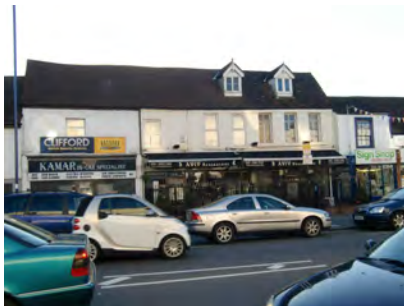
Picture 5.40 No. 85-89 High Street - likely to date to the 18th century with timber framing hidden behind render facing
