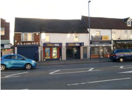
Picture 5.21 Nos. 81-85 High Street, Edgware illustrate the attractive rustic appearance of buildings along the High Street which signage currently does not enhance
