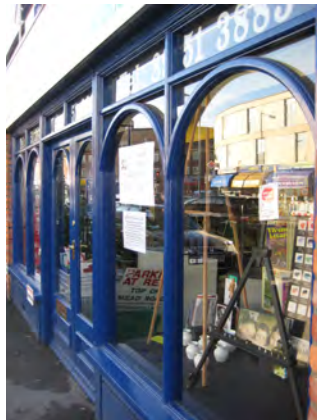
Picture 5.63 Attractive timber shopfront to no. 91 High Street, Edgware is an asset within the Conservation Area
