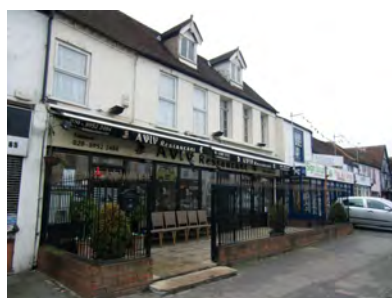
Picture 5.73 Front boundary to nos. 87-89 High Street, Edgware
