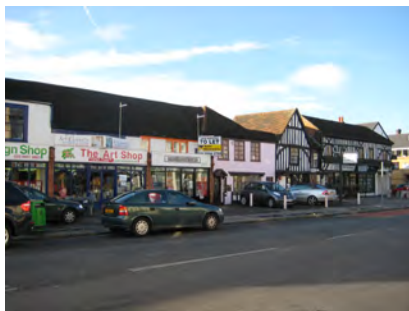
Picture 5.15 View westwards along the High Street illustrating the high density, small scale, linear terraced development that characterises the Conservation Area
