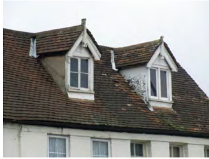
Picture 5.50 Dormer windows at nos. 87-89 High Street, Edgware
