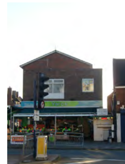
Picture 5.69 Railings around the corner of Edgware Road and Whitchurch Lane are damaged and add clutter to the streetscene
