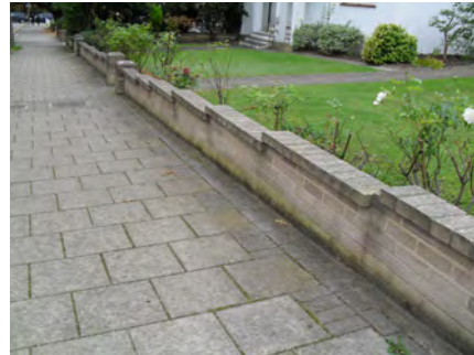
Picture 4.97 Original low boundary treatment to number 5 Kerry Avenue looking southwards
