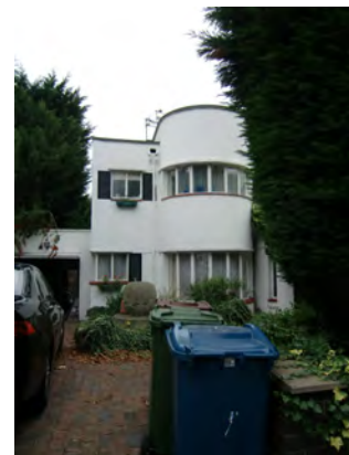
Picture 4.60 View towards 4 Kerry Avenue today
