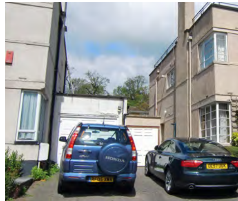
Picture 4.92 Garages between numbers 4 and 6 Valencia Road, number 4 with the original sundeck feature above
