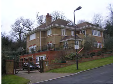
Picture 4.70 Kerry House Flats
