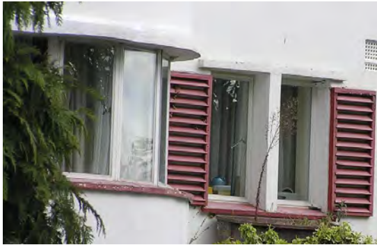
Picture 4.80 Vertical emphasis of Crittall windows along Kerry Avenue, at 4 Kerry Avenue, and right at 5 Kerry Avenue
