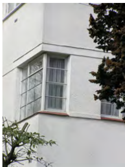
Picture 4.78 Crittall windows sometimes follow the sharp corner of a building to emphasise the strong geometrical forms as above, and in the picture right, on 2 Valencia Road
