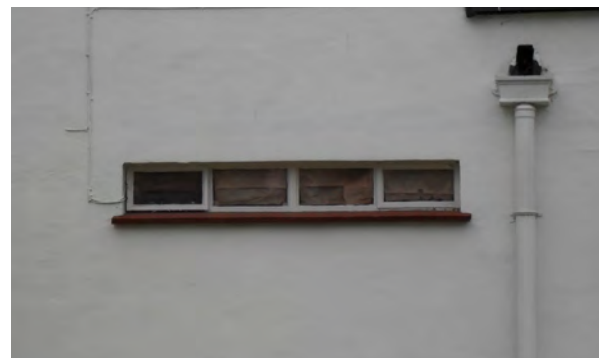
Picture 4.83 Flat window on number 5 Kerry Avenue
