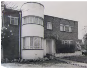
Picture 4.52 1 Kerry Avenue before it was fully rendered and partly extended (date unknown) Source: Local history library.
