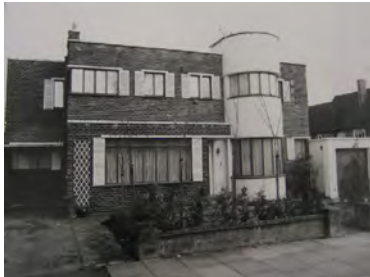
Picture 4.57 Number 2 Kerry Avenue before some of the modern alterations to the building (date of photo unknown) Source: Local history library
