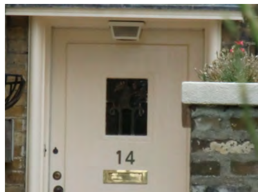
Picture 4.67 Important original detail - New Zealand rabbit in glass of the front door of 14 Kerry Avenue
