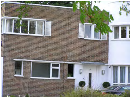
Picture 4.74 Exposed brickwork on the original 1930s Modernist buildings
