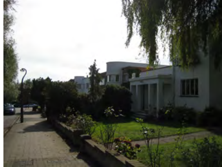
Picture 4.28 Softly landscaped gardens on the western side of Kerry Avenue
