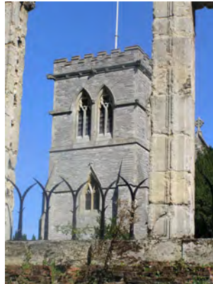
Picture 3.35 View of the battlemented tower of the grade II* St John the Evangelist from within the Old Stanmore Church. This tower forms the source of numerous key views.
