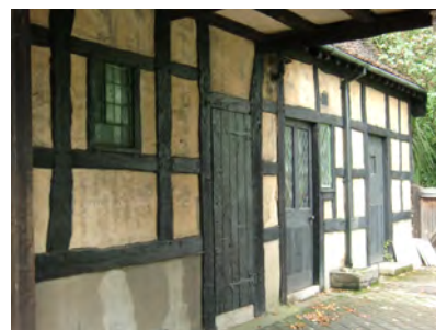
Picture 3.49 Lathe and plaster infill on wall to the grade II listed Cowman's Cottage, Old Church Lane and part of its roof over the carriage-way
