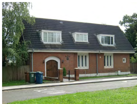
Picture 3.22 The Old Station fronting mini Green, junction of Gordon Avenue and Old Church Lane
