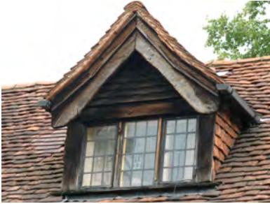
Picture 3.70 Small pitched roof dormer on Church House Cottage, Old Church Lane
