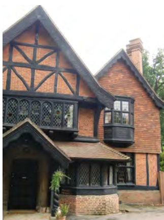
Picture 3.43 Varied roofscape, decorative mock timber framing, tile hanging and jetty overhang
