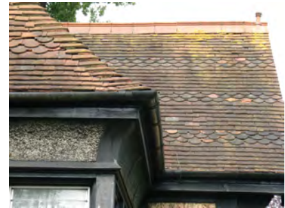
Picture 3.39 Good decorative tile roof
