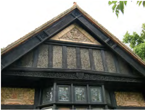
Picture 3.38 Decoratively carved timber work to gable end with delicately carved terracotta panel and stone mullioned windows within
