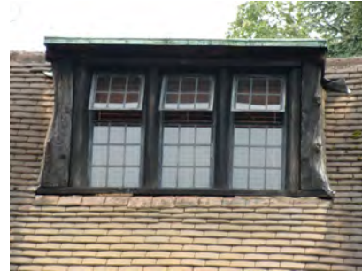
Picture 3.71 Sloping pitched roof dormer to the Tithe Barn, Old Church Lane
