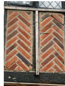
Picture 3.67 Herring bone patterns infilling mock timber framing panels on the locally listed Gate House Lodge, Old Church Lane
