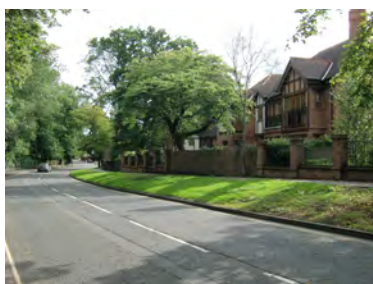
Picture 3.94 Important grass verges along Old Church Lane, here near Kestrel Court
