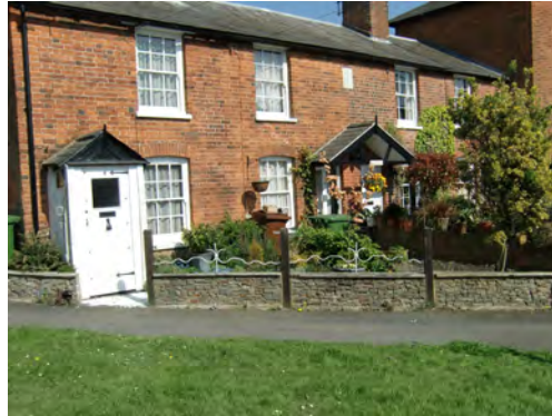
Picture 2.55 Pinnacles Place, Green Lane
