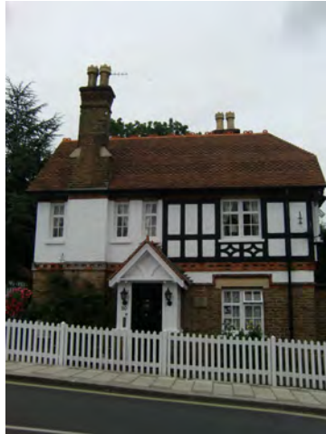
Picture 2.44 Locally listed, The Cott, no. 80 Stanmore Hill
