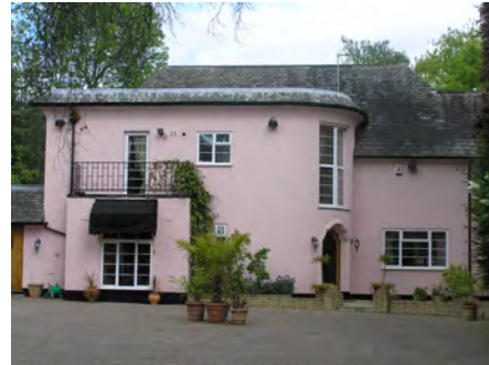
Picture 2.23 Modernist property, lower reaches of Green Lane
