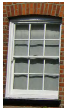
Picture 2.89 Six over six pane timber sash window
