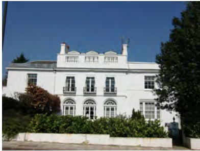
Picture 2.33 Grade II listed Goodengate, Stanmore Hill
