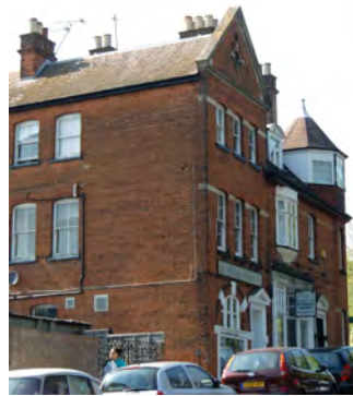
Picture 2.29 Landmark building within the upper reaches of Stanmore Hill
