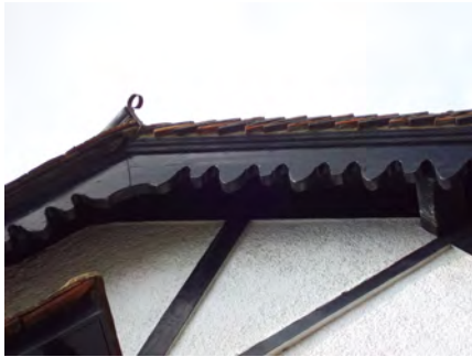
Picture 2.64 Decorative timber bargeboard on the Tudor Revival style 129 Stanmore Hill
