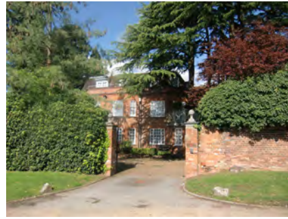
Picture 1.48 Good brick boundary wall to Wellington House
