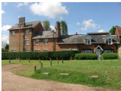
Picture 1.14 Side of 11 Little Common (Woodbine Cottage)
