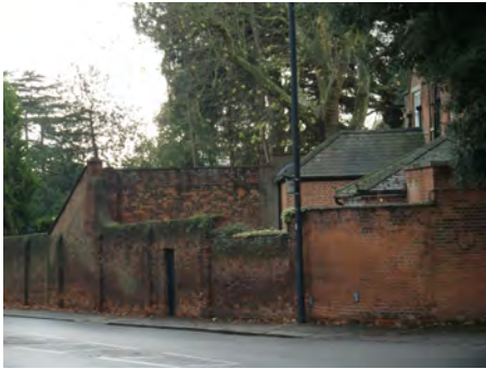
Picture 1.47 Listed wall to Hill House
