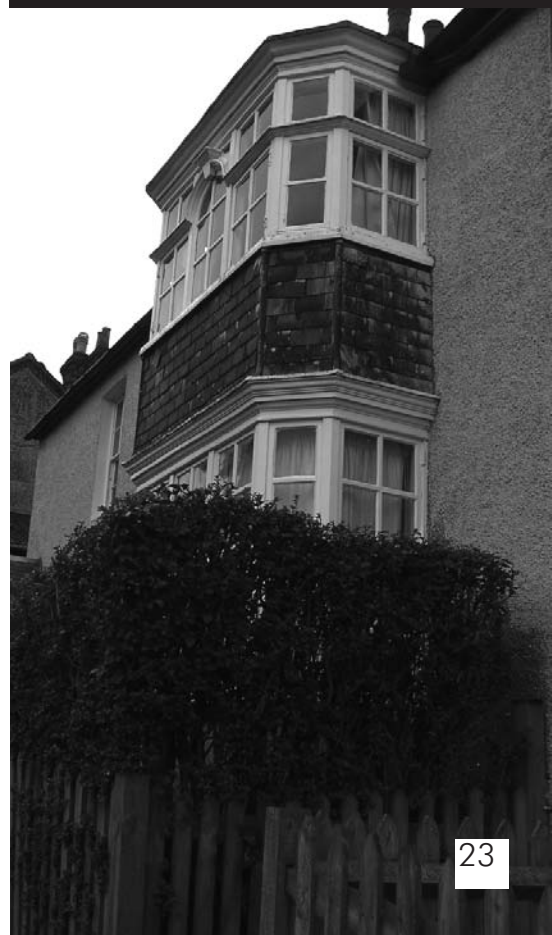
Cricket Field Cottage, Middle Path: Attractive Two Storey Casement Window With Grey Tile Hanging
