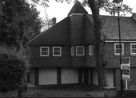
Arts and Crafts inspired tile hanging detail of number 21 Byron Hill Road
