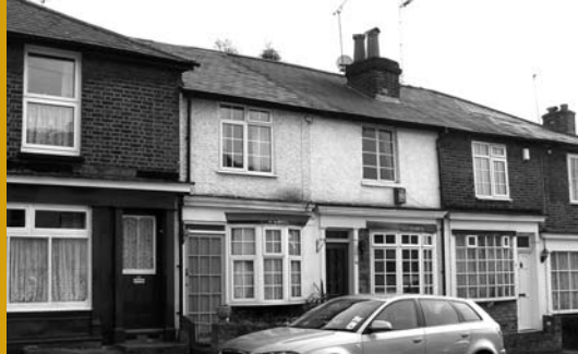
Base of Middle Road: Shops converted to residential use in the mid C20th leaving shopfront remains clearly visible
