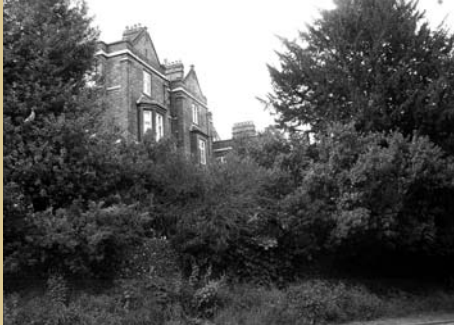
Rear of Boarding houses on Grove Hill
