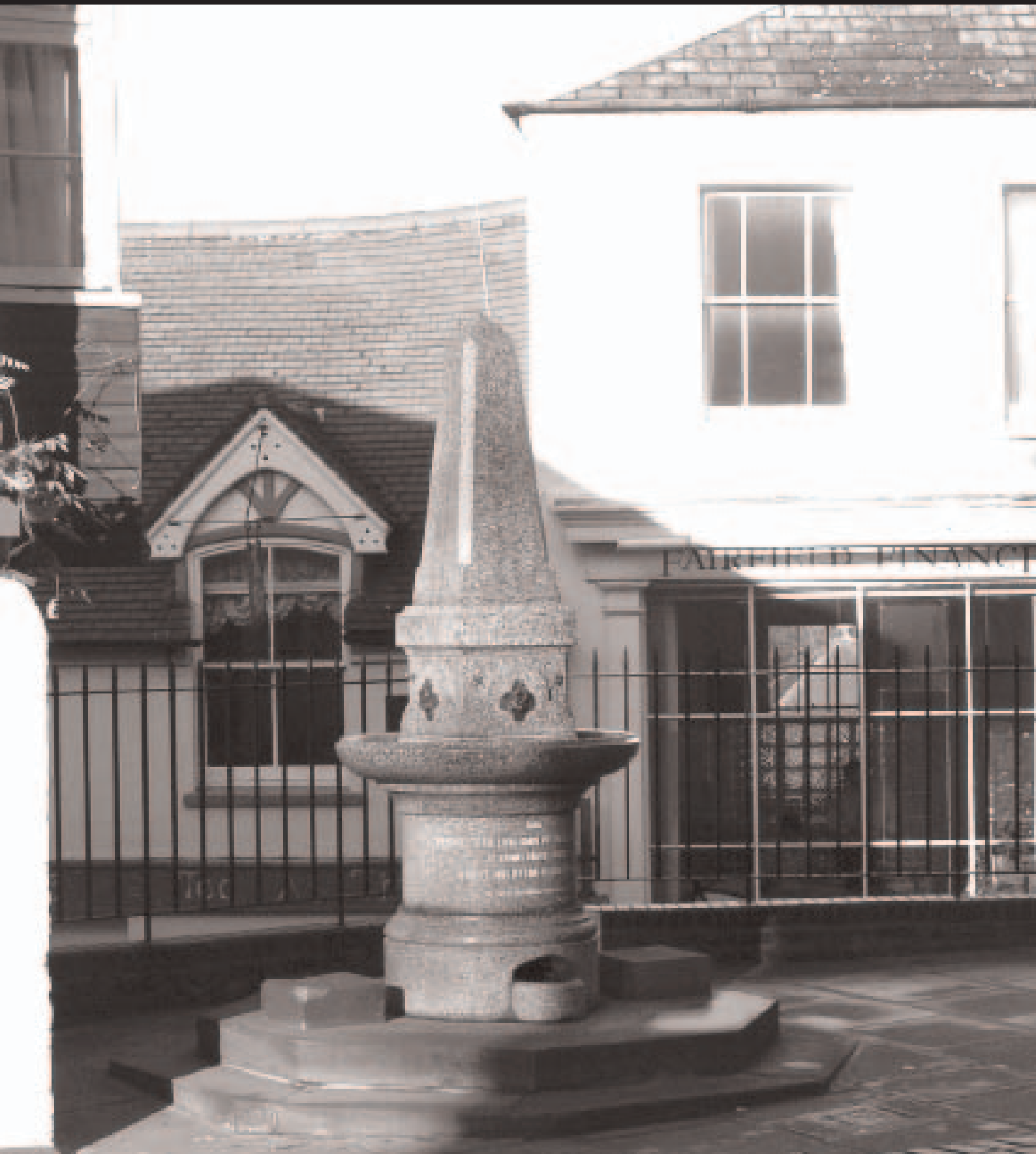
The restored Fountain, on the High Street at the junction of West Street
