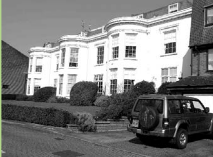
21 Harrow Fields gardens - bow-bayed Regency buildings
