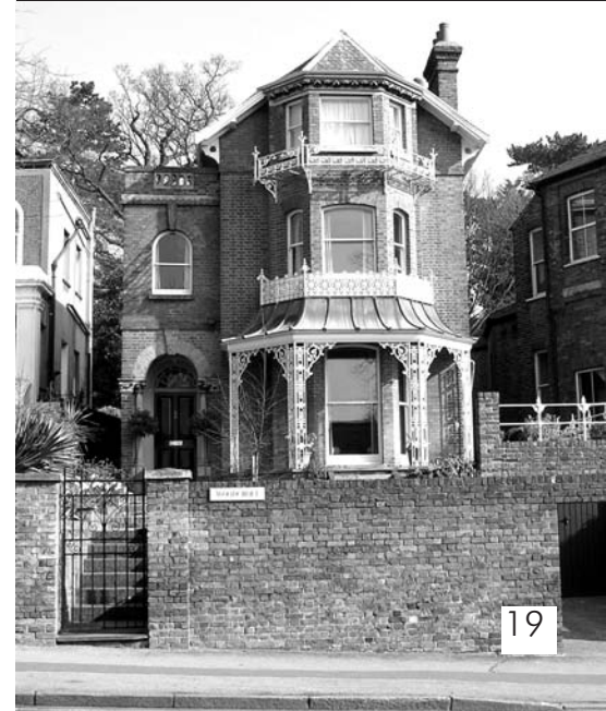
Decorative ironworks, a key feature of many larger, classically inspired Victorian buildings
