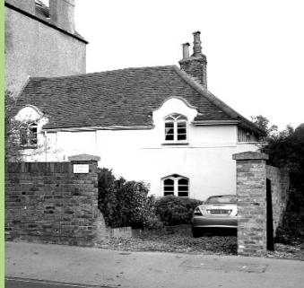
Toll Gate Cottage - thought to have originally been a Coach House
