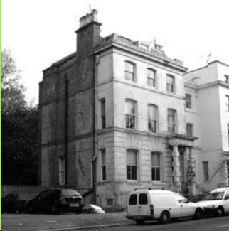
Properties in a poor state of repair
