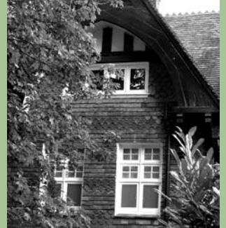
Tile hanging is a predominant architectural feature of the area. Here it is at Egerton
