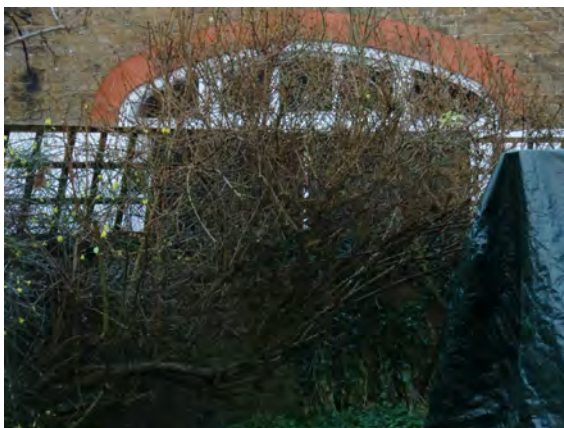
Picture 1.28 Central gauged red brick arch
