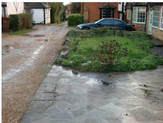
Picture 1.55 Absence of front boundary treatments helps preserves the informal, semi-rural character
