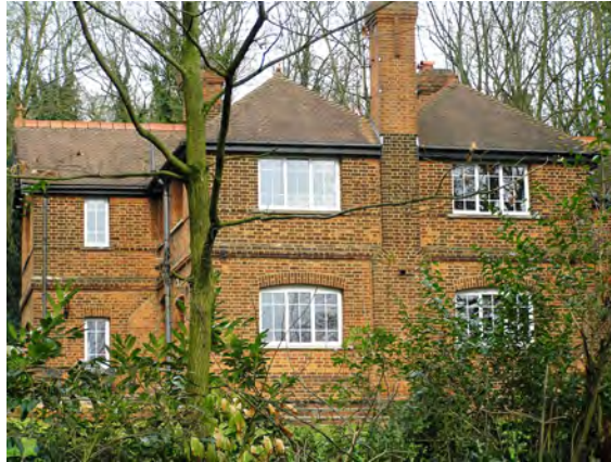
Picture 1.8 3&4 The City, Old Redding before a recent fire which part destroyed the building
