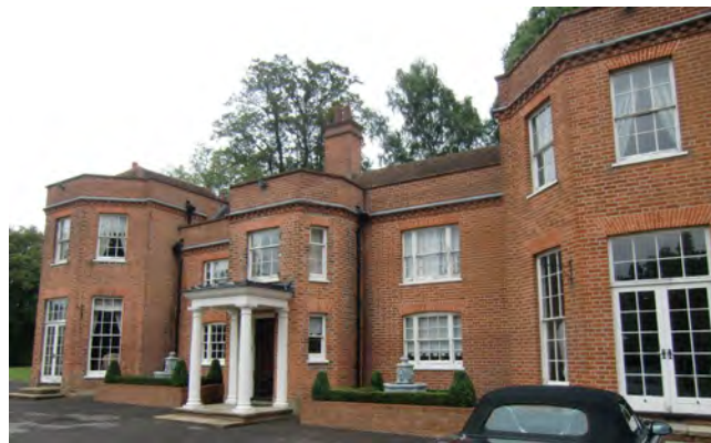
Picture 1.21 The Kiln house provides an architectural focal point
