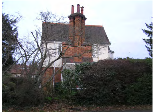
Picture 1.14 Decorative chimney in an Arts and Crafts style
