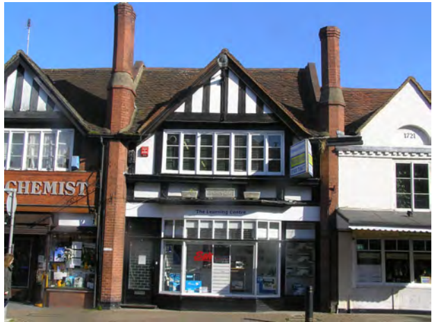
Picture 3.56 Timber shopfronts
