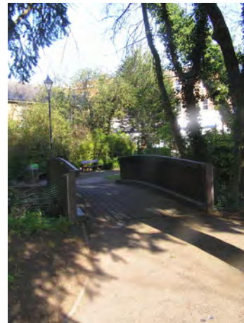
Picture 3.39 Bridge over the River Pinn
