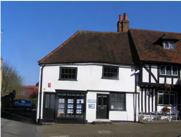
Picture 3.6 16th Century timber framed core beneath modern tiles and re-plastering
