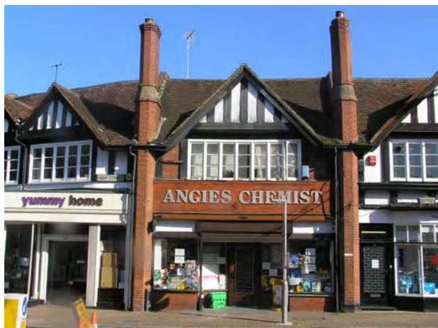
Picture 3.47 Traditional shopfronts
