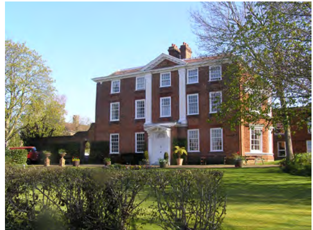
Picture 3.30 Pinner House, dates from 1721, with pediment doors case, fluted Ionic pilasters and fanlight
