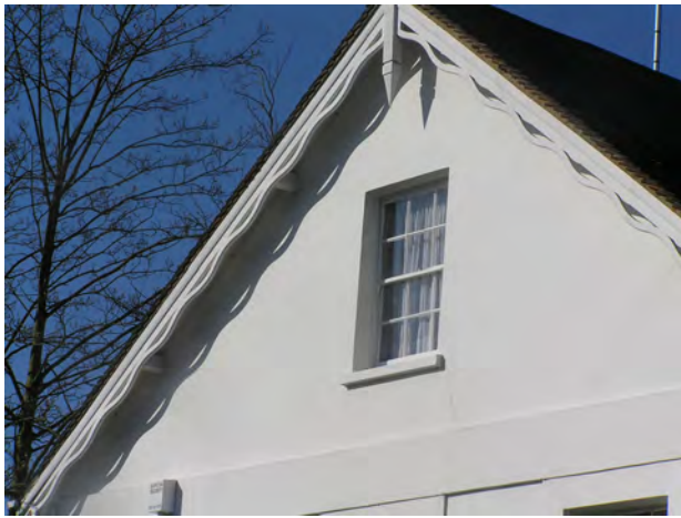
Picture 3.17 Decorative eaves on Paines Lane
