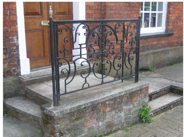
Picture 3.35 Decorative wrought iron railings
