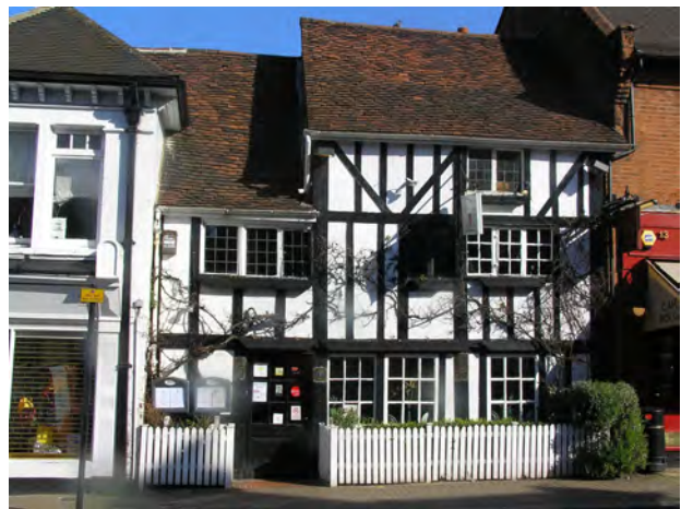
Picture 3.4 Early 16th Century timber framed building
