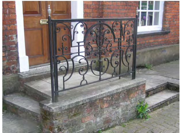
Picture 3.35 Decorative wrought iron railings
