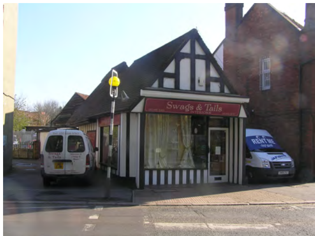
Picture 3.51 Simple painted fascia boards
