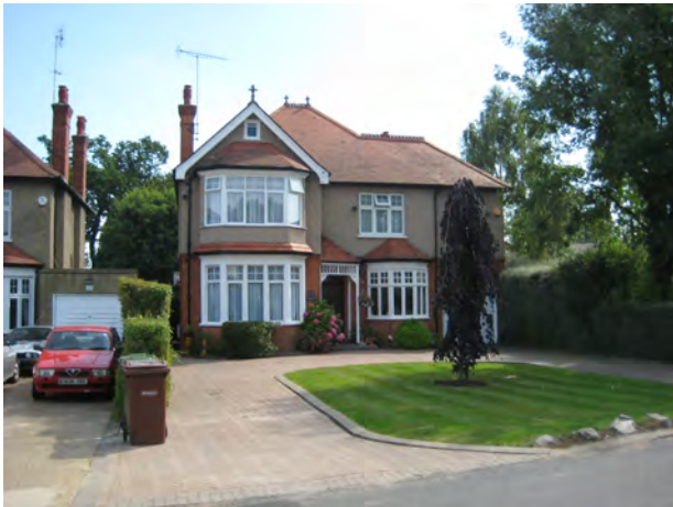
Picture 4.25 The contrast between original and replacement windows is evident
