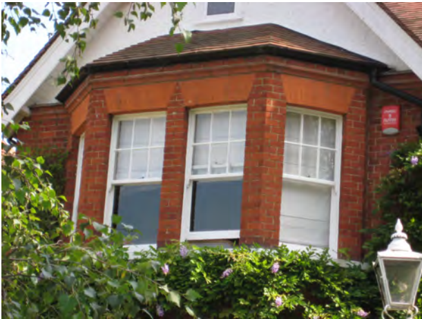
Picture 4.29 Gauged brick arches
