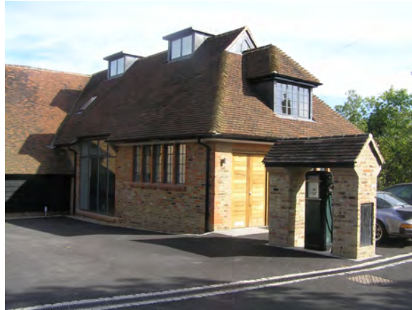
Picture 5.19 Pump House
