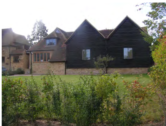
Picture 5.18 Rear of East Barn and the Pump House
