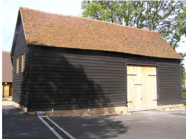
Picture 5.15 Front of North Barn
