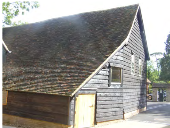
Picture 5.16 Side and rear of North Barn
