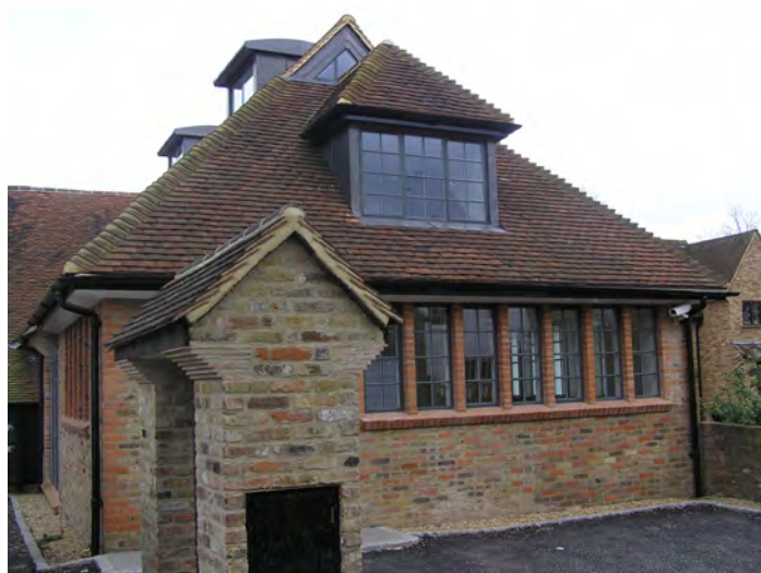
Picture 5.3 Former barn dating from 1953, now Pump House
