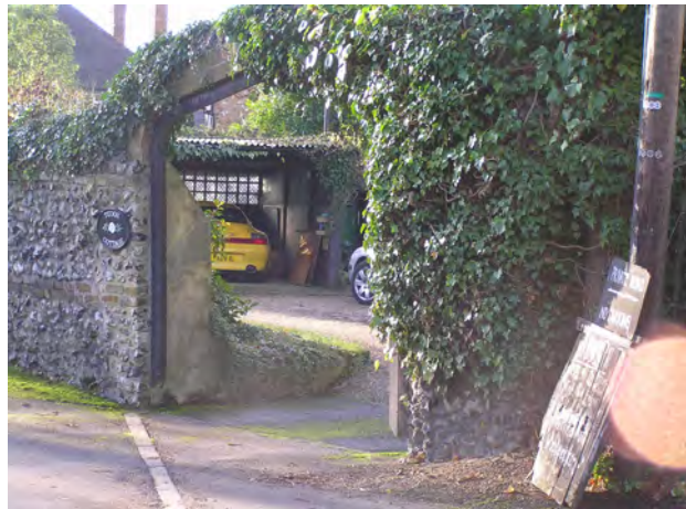
Picture 5.28 Flint wall
