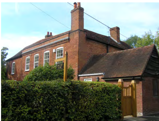
Picture 5.13 Important View Towards East End House
