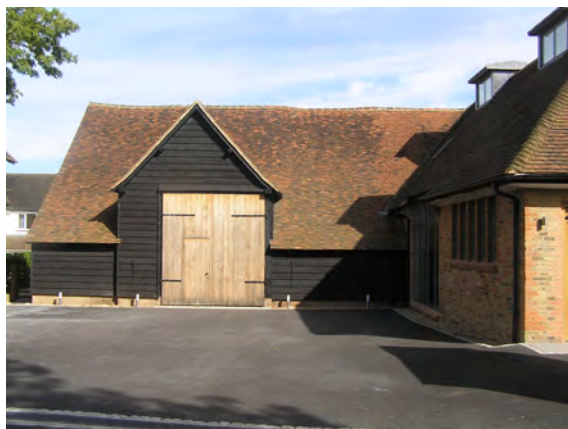
Picture 5.17 Front of East Barn
