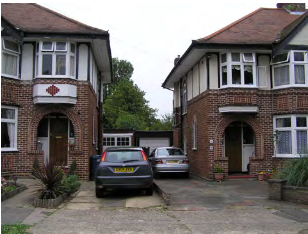
Picture 6.22 Roof profile and garages
