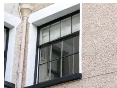
Picture 7.42 Original timber window
