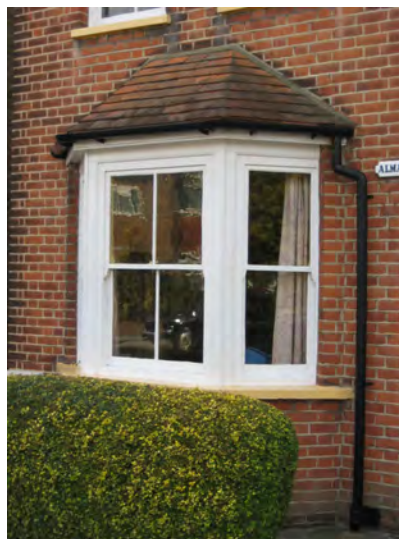
Picture 7.31 Elegant, simple ground floor timber bay window
