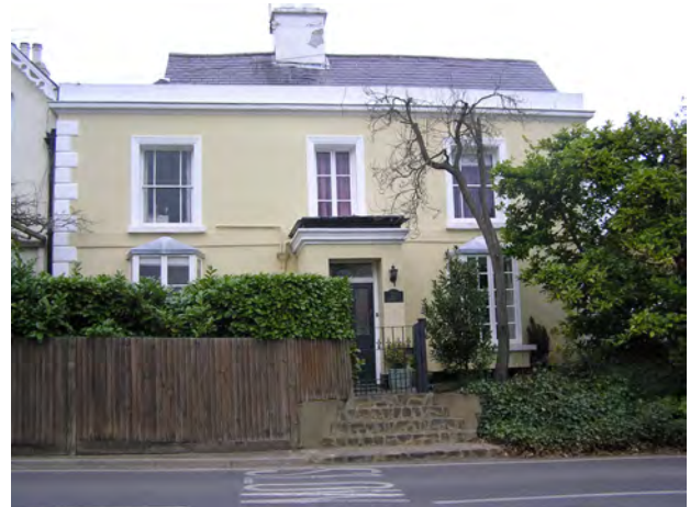
Picture 7.20 Timber framed with Georgian brick infill
