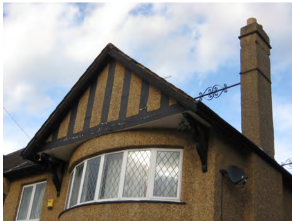
Picture 7.27 Gable end with mock Tudor detailing, Cecil Park
