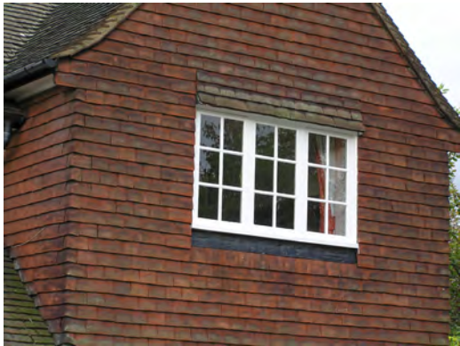
Picture 8.31 Tile hung gable frontage at Woodhall Gate
