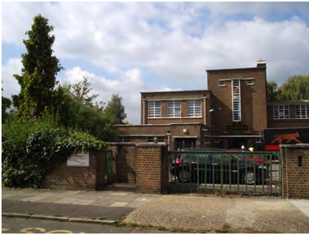
Picture 8.14 Pinner Wood School is a 1930s building with simple and elegant clean lines in the Art Deco tradition.
