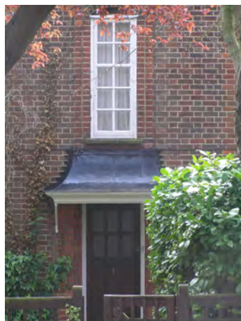
Picture 8.26 Original door
