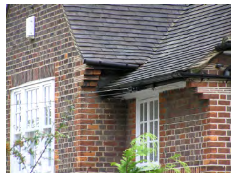
Picture 8.30 Corbels jut out under eaves
