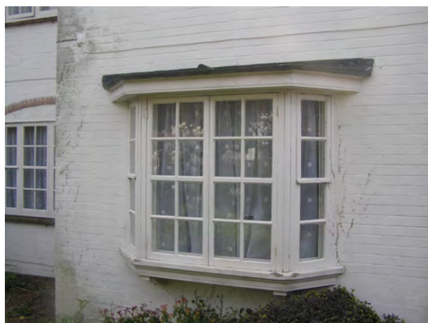
Picture 8.22 Casement box bay with lead flashing
