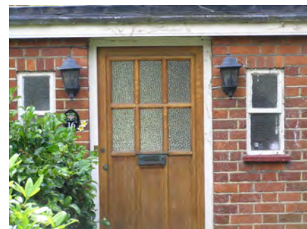
Picture 8.27 Small windows set either side of doorway
