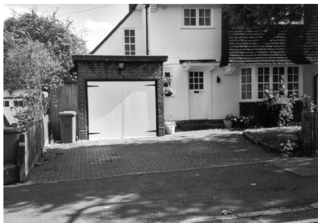
An example of inappropriate 'hard' frontage
