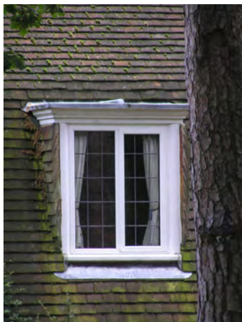
Picture 9.39 Box windows
