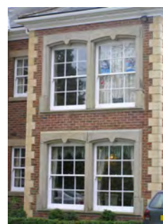
Picture 9.36 Stone quoins and window surrounds
