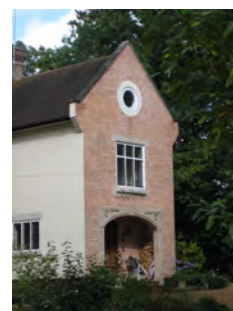
Picture 9.27 Stone lintels
