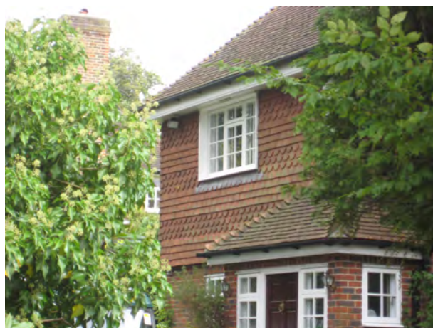
Picture 9.13 Tile hanging
