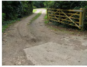
Picture 10.32 Timber 5 bar gate
