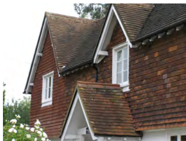
Picture 10.23 Gable ends
