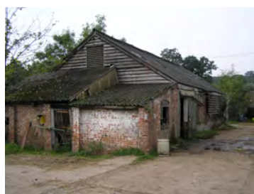
Picture 10.25 Former granery
