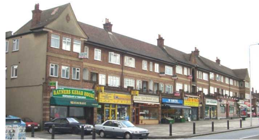
Picture 11.14 Simple traditional shopfronts with narrow fascias
