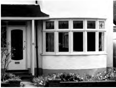
Picture 12.14 Bay windows and leaded lights
