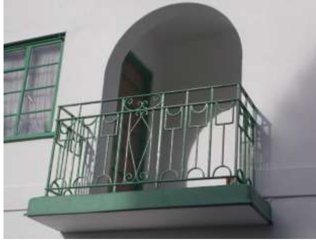
Figure 87: Painted finish to the balconies link in with the window finish
