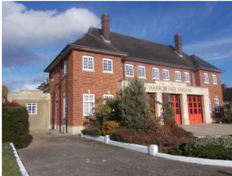
Figure 12: Pinner Fire Station built 1937
