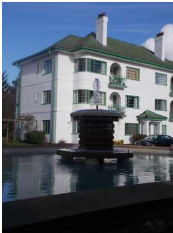
Figure 59: The geometrically designed ornamental garden to Pinner Court, with listed fountain centrepiece, complements the Art Deco building
