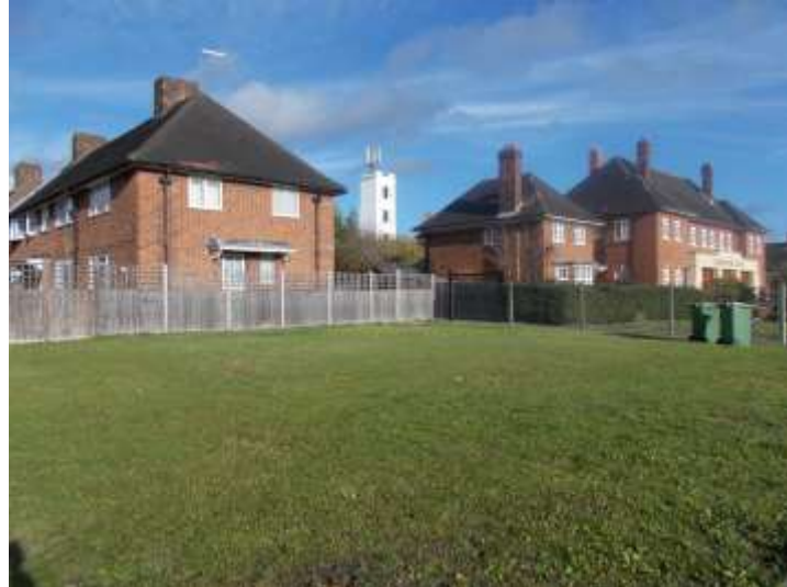
Figure 60: Pinner Fire Station, training tower and cottages form the only known example of an inter-war fire station complex in Harrow
