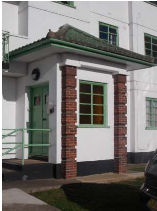
Figure 44: Typical Art Deco style hipped green pantile roof with oversailing sprocketed eaves and exposed brickwork columns to the porches to Capel Gardens
