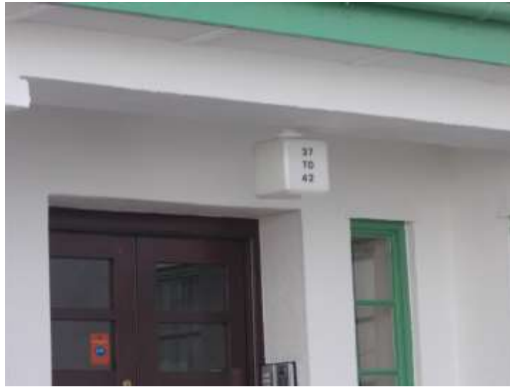
Figure 57: Cube shaped light above the entrance doors to the Pinner Court flats are an important part of the Art Deco design.
