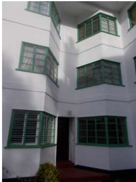
Figure 79 and 80: Typical Crittall windows on Pinner Court
