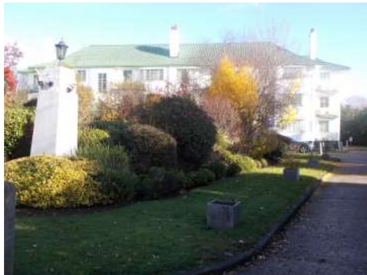
Figure 56: One of two Art Deco/Modernist style lamp standards to Capel Gardens forming part of the geometrically planned landscaping
