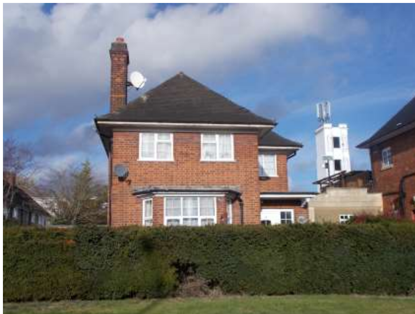
Figure 69: Cottage 18 with fire tower to the rear
