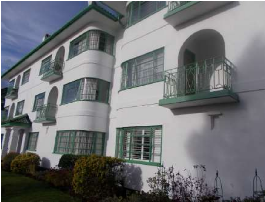
Figure 45: Curved corner bay windows feature on Pinner Court (above) and Capel Gardens being an important Art Deco feature
