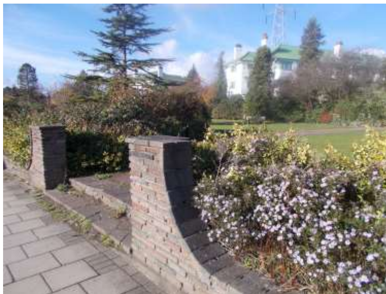
Figures 91 and 92: Low brick walls form important boundary treatments to boulevard gardens
