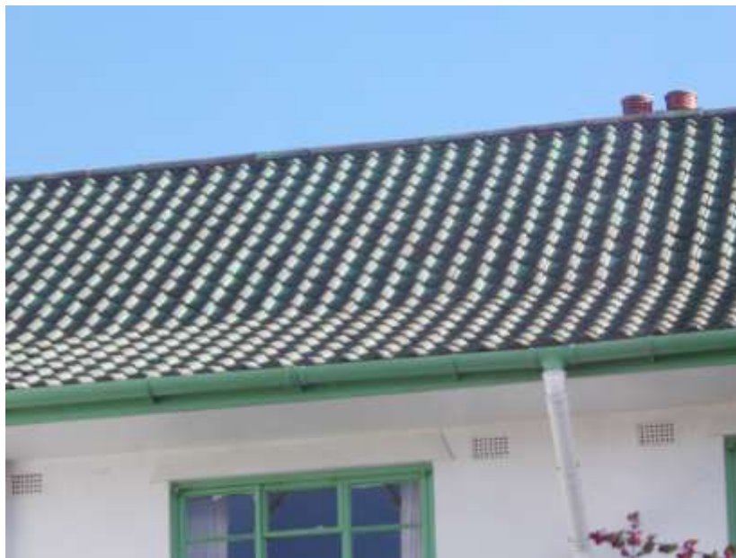
Figure 49: Typical pan tiled hipped roofs with sprocketed eaves of Capel Gardens
