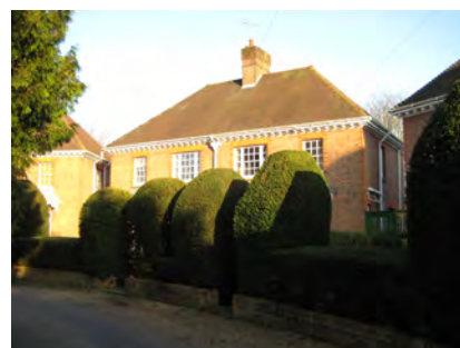
Picture 2.11 Hipped roofs and centrally located chimneys
