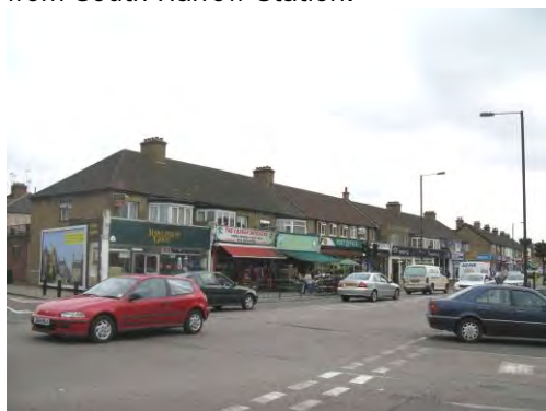
South side of Northolt Road, from junction with Eastcote Lane.
