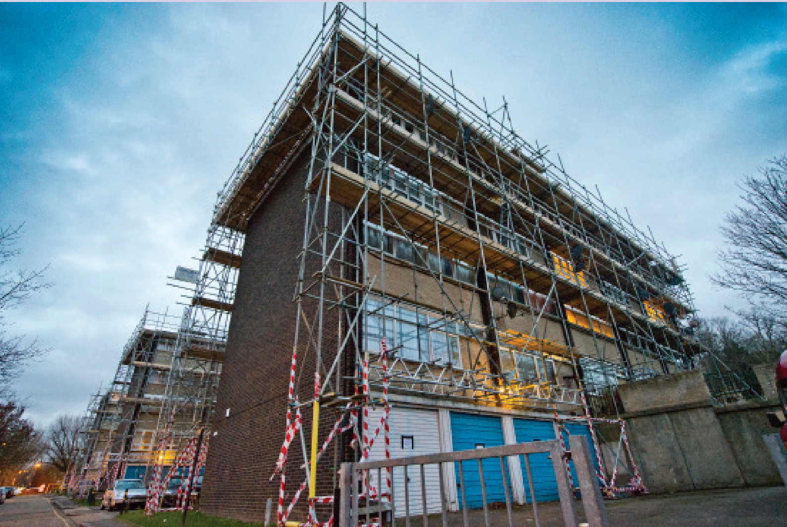
Northolt Road refurbishment
