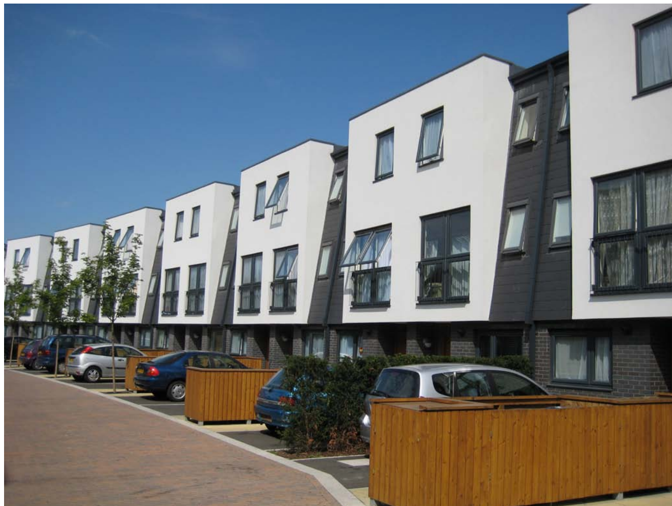
Picture 8 Affordable Housing at Honeypot Lane
