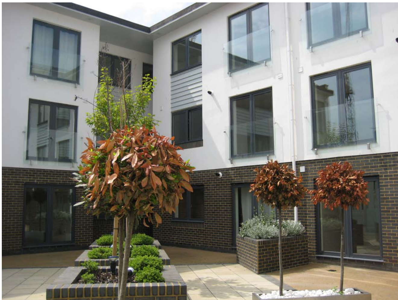
Picture 7 High Density Development on Pinner Road
