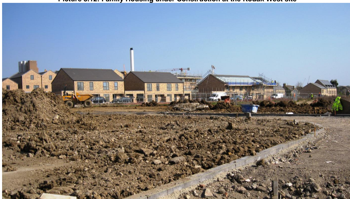
Picture 3.12: Family Housing under Construction at the Kodak West site
