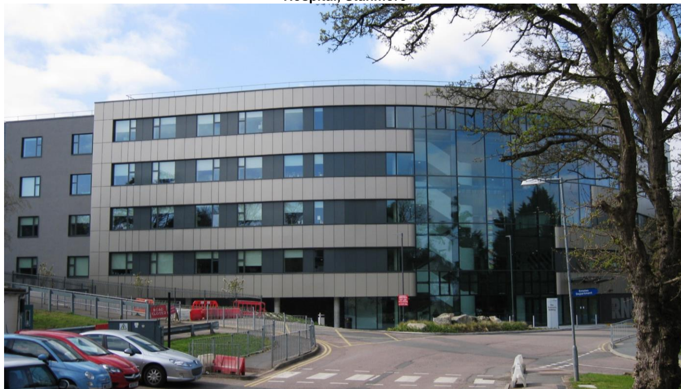
Picture 3.2: New Inpatient Accommodation Block at the Royal National Orthopaedic Hospital, Stanmore
