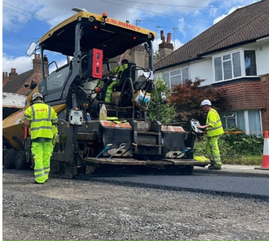
We resurfaced more than 60 roads and paths
