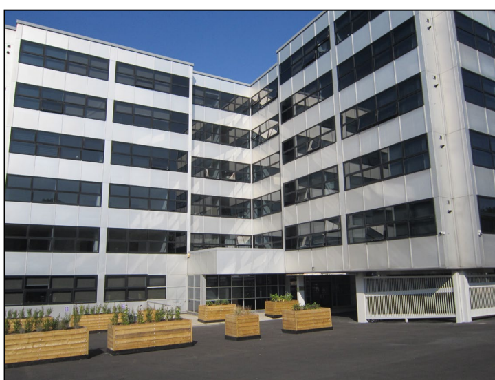
Bovis House, 142 Northolt Road, South Harrow
