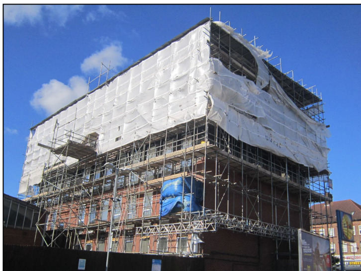
Kajaine House, 57-67 High Street, Edgware
