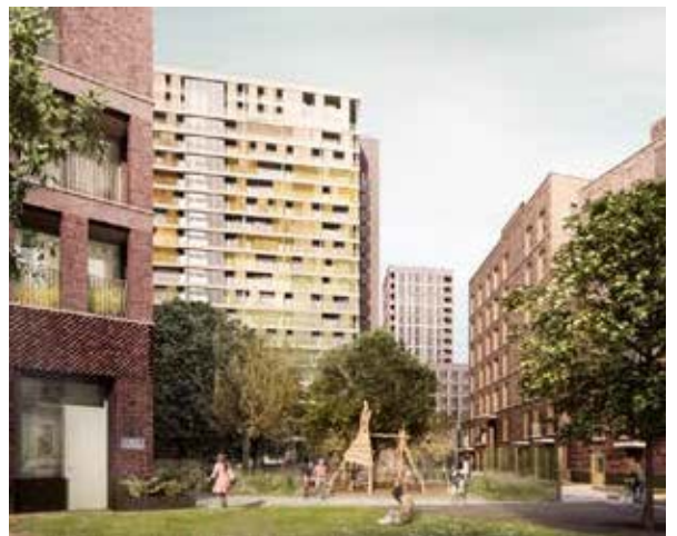
Agar Grove is a high density mid/high-rise Passivhaus development promoting a 'fabric-first' approach to energy performance and human comfort
