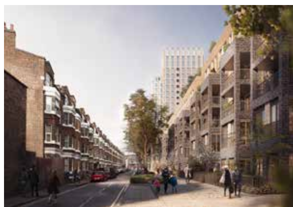
Proposed new build scheme of six storeys in a suitable-and-sensitive location, where the lower four storeys (R) reinforce the scale of existing buildings across the street (L) while the upper two floors stepped back from the street. Further in the background, a tower is proposed in a more central and suitable location next to a station.
