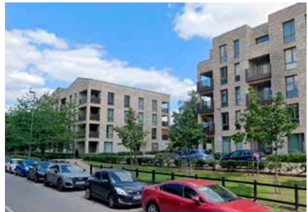
Stepping up in scale along the A5 corridor on the Brent side
