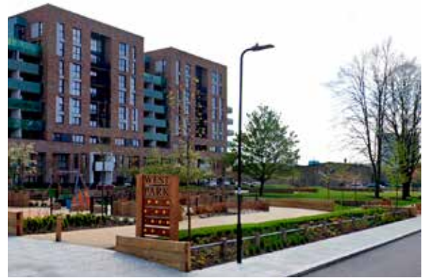
High density, 10 storey perimeter blocks form a part of the Acton Gardens masterplan, Ealing, which includes an extensive open space network comprising three public parks, communal gardens, green streets and allotments.
