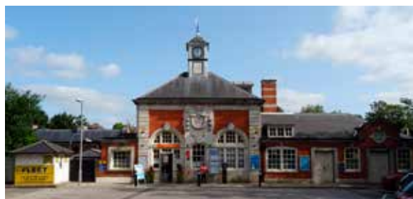
Hatch End station is a heritage asset that serves its community well but could see its setting enhanced through public realm improvements and mixed uses.
