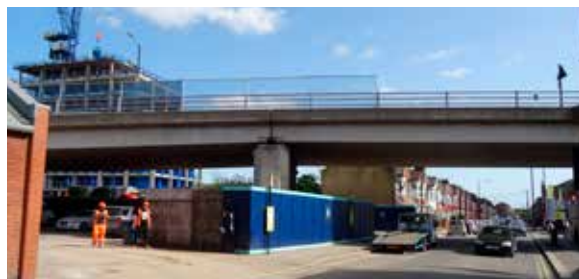
A409 flyover Masons Avenue, Wealdstone. The level change and major infrastructure creates an illegible environment and poor sense of place.
