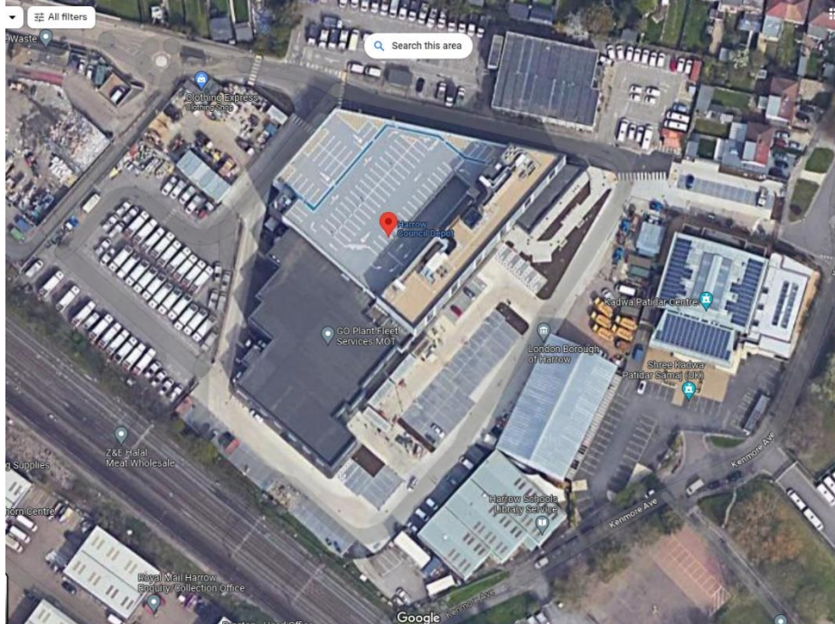
Figure 4.3: Satellite view of Harrow Council Hub, the car park for fleet and staff vehicles.
