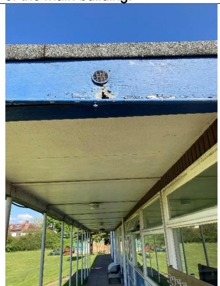
Photograph 6. PRF into roof cavity / eaves of south side of main building.
