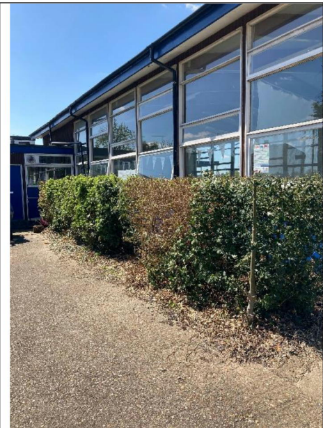
Photograph 1. Ornamental hedge on east side of main building.
