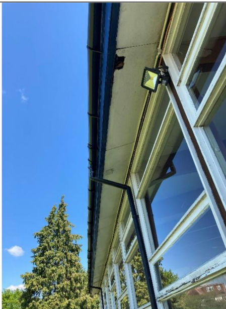
Photograph 2. PRF on eaves of west side of main building.
